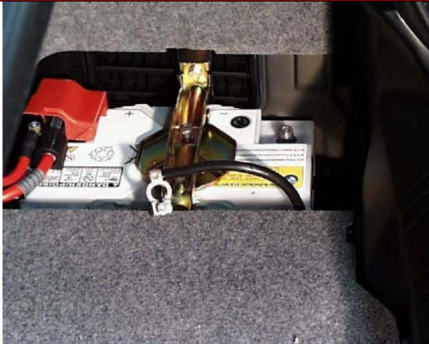
Figure 1 Disconnect the Negative terminal on the battery.
