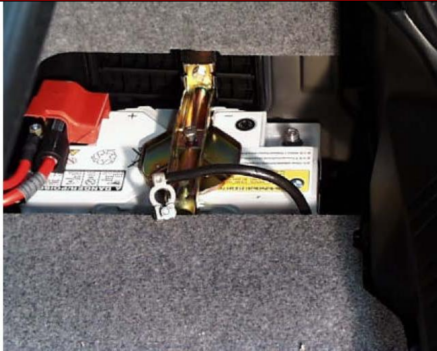
Figure 1 Disconnect the Negative terminal on the battery.
